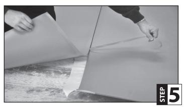
**Step 5:**Remove the adhesive liner and adhere the foam to the film overlap.
